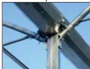
arc-column connection
