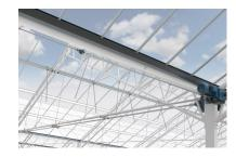
Controlled ventilation is essential for an optimal climate in wide-span greenhouses. Ventilation is realised by means of continuous windows in the ridge of the greenhouse. We have the knowledge, expertise and extensive product range to contribute to an optimal climate for the best results
