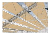
The use of (roof roll) screens in wide-span greenhouses not only protects the plant from harmful sunlight, but they also have the ability to reduce light and save energy by retaining heat. In this way, screens contribute to the sustainability goals. To make this possible, we offer a wide range of drives that have been specifically developed for this purpose.
