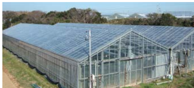
60μm thick F-Clean® installed in the Aichi region of Japan in 1988 (photographed 2009)
