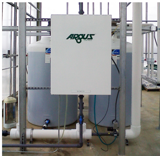
Argus A/B in-line injection system using two stock tanks
