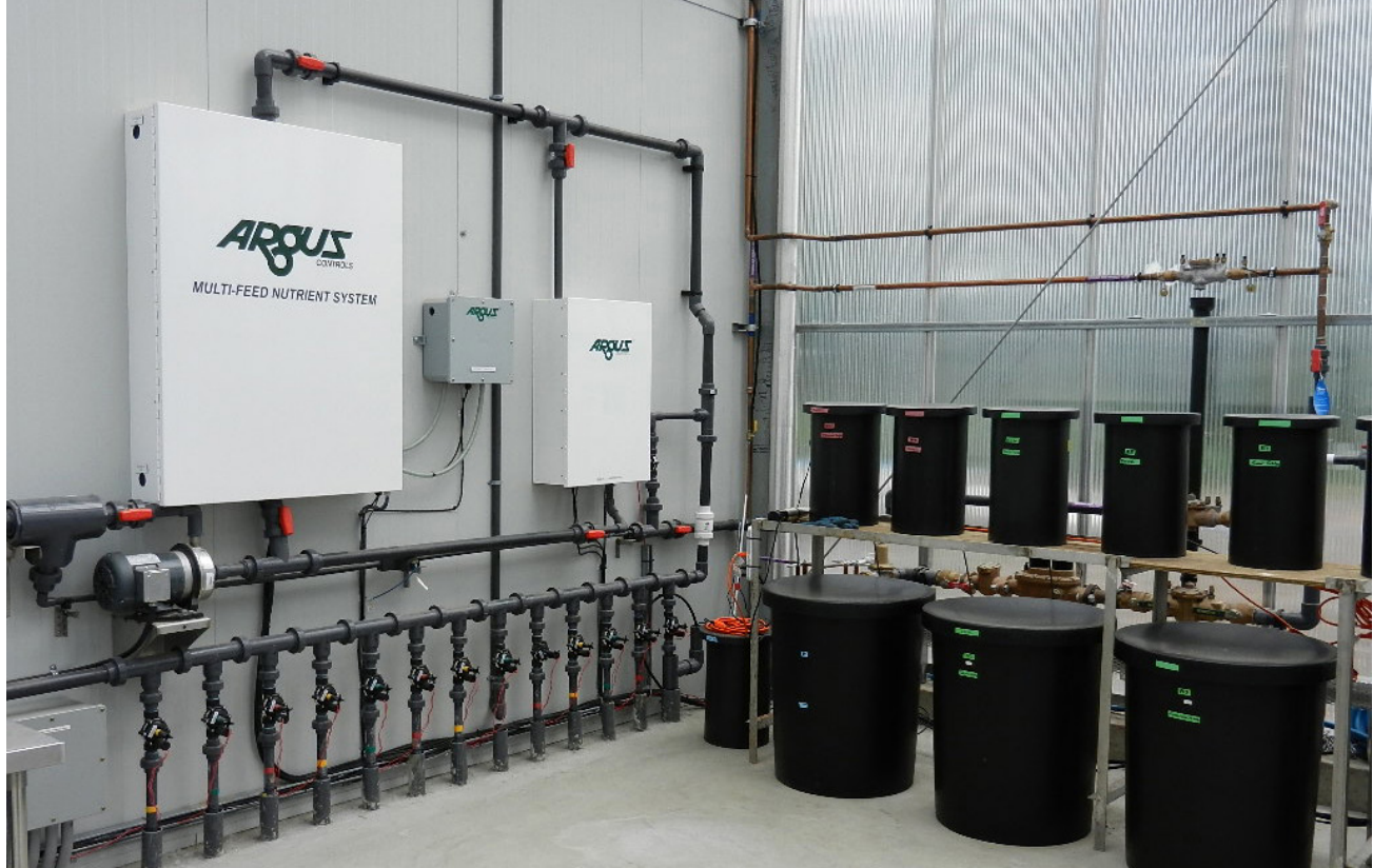
Single-element nutrient dosing system
