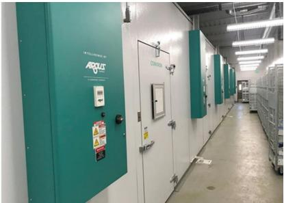
Conviron's Cannabis One<sup>™</sup> drying rooms are sized to suit a range of spaces and are compatible with any drying cart or rack used with dry- or wet-trimming processes. Multiple rooms can be installed to match the cultivator's harvest and production schedule.
