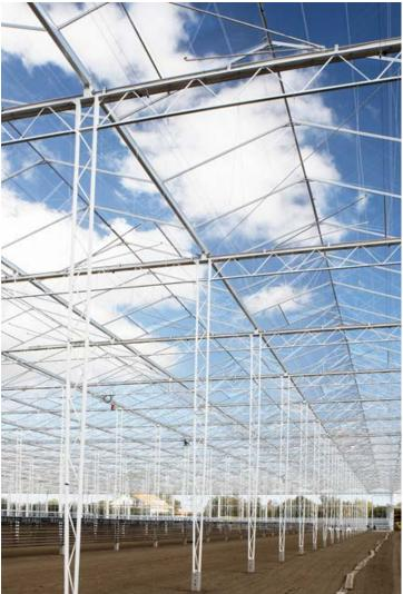
That we are flexible and always looking for ways to optimize our greenhouse systems is proven by the introduction of our Twinlight® column. The Twinlight® column is an open column which consist of less steel and enables the sun to shine through.
